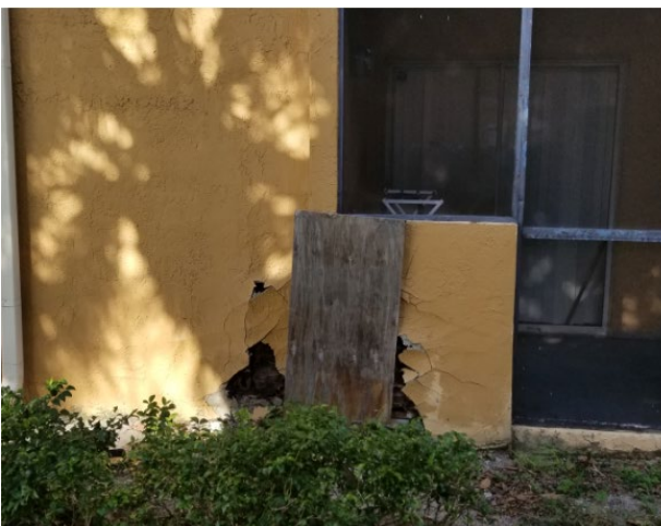
Photograph 11: Opening in the exterior wall
