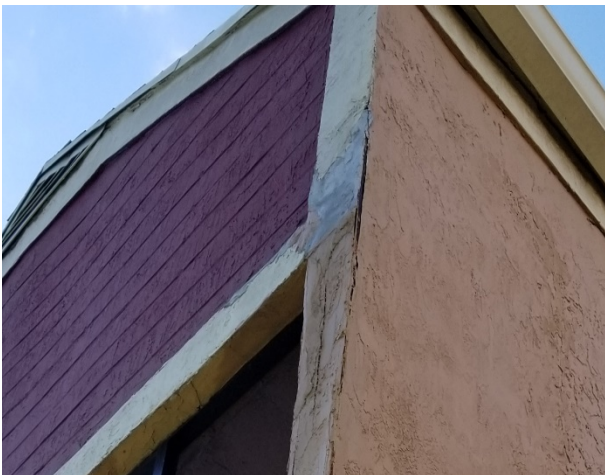
Photograph 11: Cracks and previous repairs on the exterior wall
