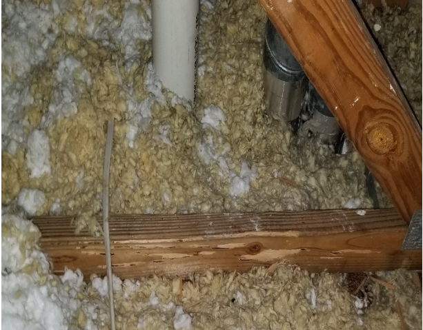
Photograph 13: Unit 204. Termites infestation and damage to bottom truss chord
