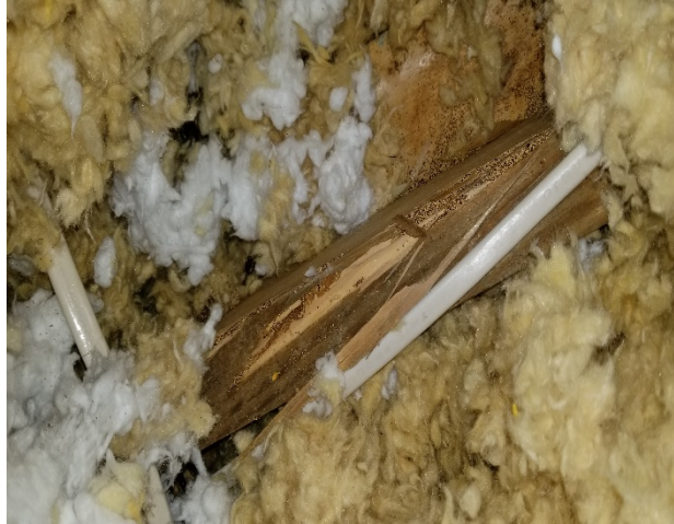
Photograph 14: Unit 207. Termites infestation and damage to bottom truss chord
