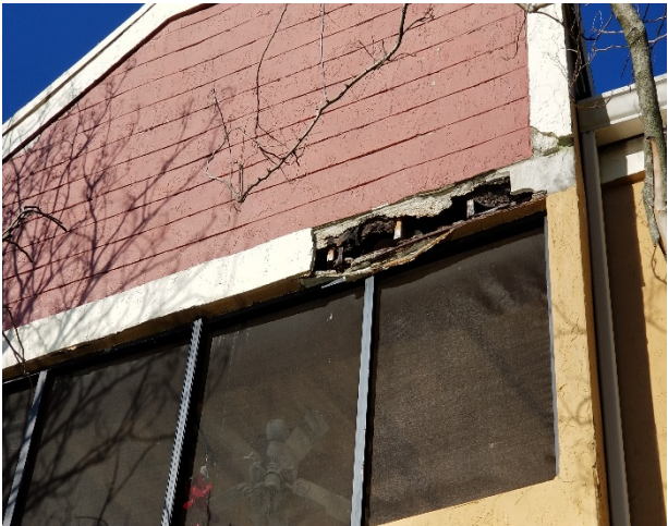
Photograph 15: Opening in the exterior wall
