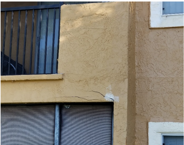
Photograph 11: Exterior wall crack
