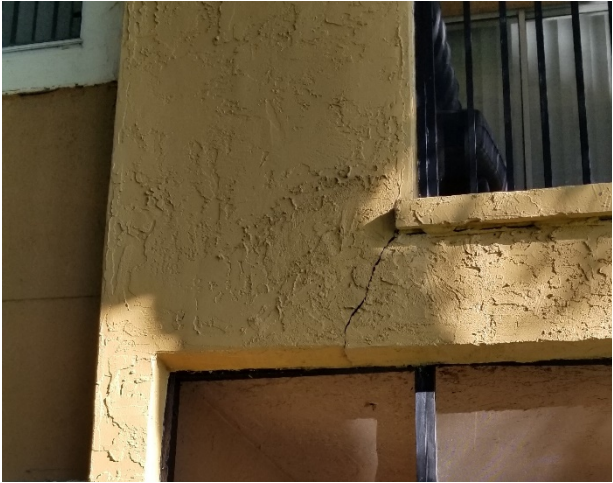
Photograph 9: Exterior wall crack
