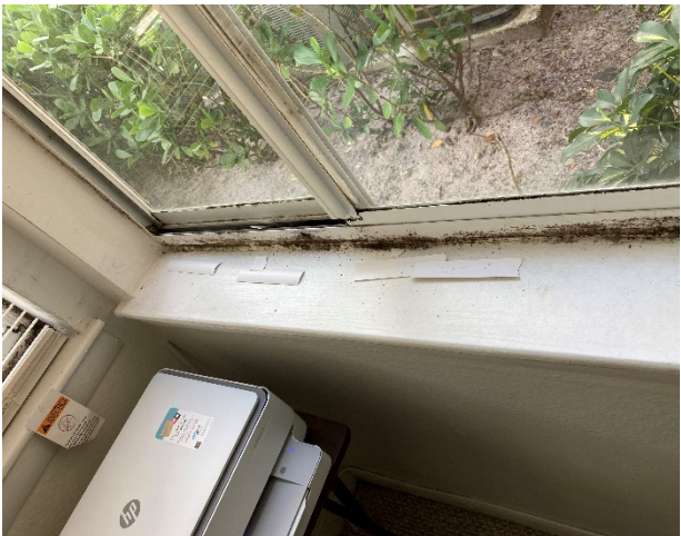
Photograph 3: Unit 104. Termites infestation and moisture damage
