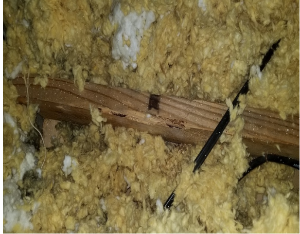
Photograph 8: Unit 207. Termites infestation
