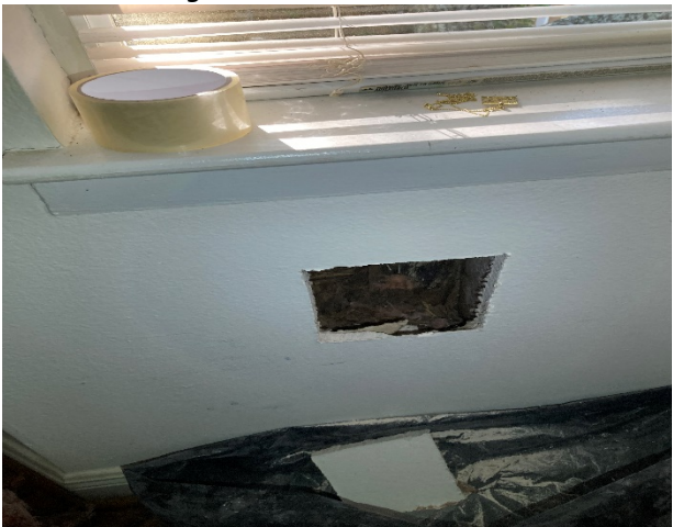
Photograph 3: Unit 104. Termites infestation and moisture damage
