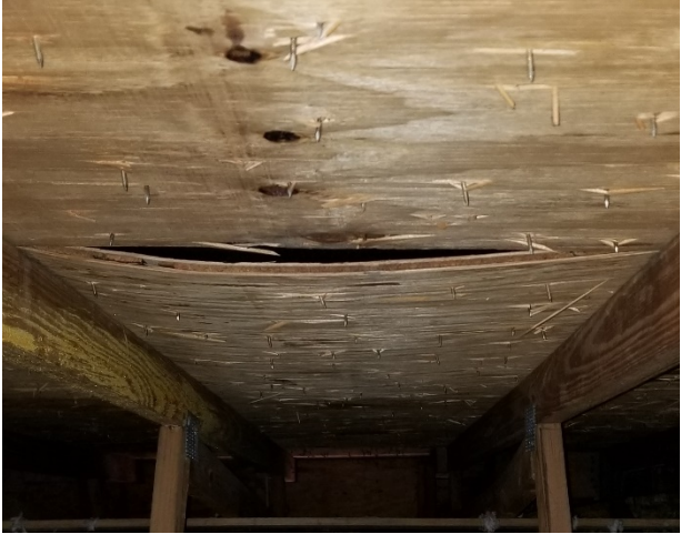
Photograph 7: Unit 205. Sagging sheathing within the attic
