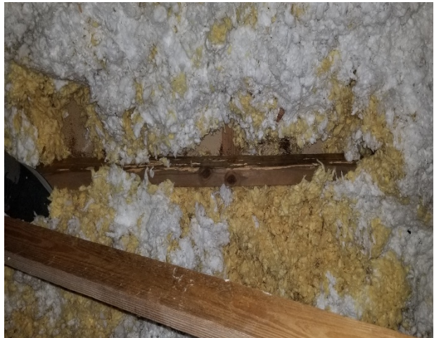
Photograph 10: Unit 206. Termites infestation and damage to the bottom truss chord
