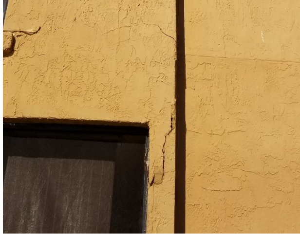
Photograph 14: Exterior wall cracks
