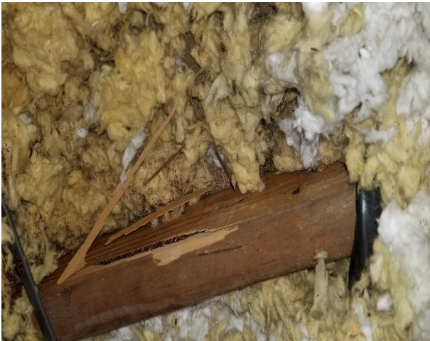
Photograph 9: Unit 201. Termites infestation and damage to the bottom truss chord
