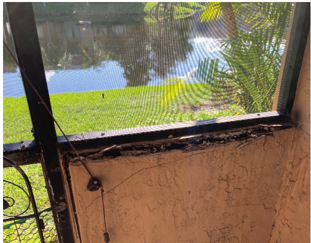
Photograph 4: Unit 108. Moisture stains and cracks within the interiors
