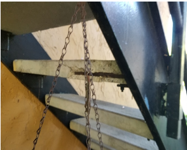
Photograph 9: Unit 201. Termites infestation and damage to the bottom truss chord
