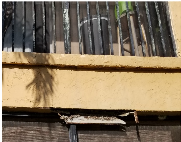
Photograph 10: Unit 206. Termites infestation and damage to the bottom truss chord
