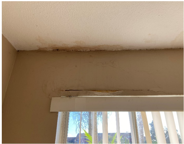
Photograph 4: Unit 108. Moisture stains and cracks within the interiors
