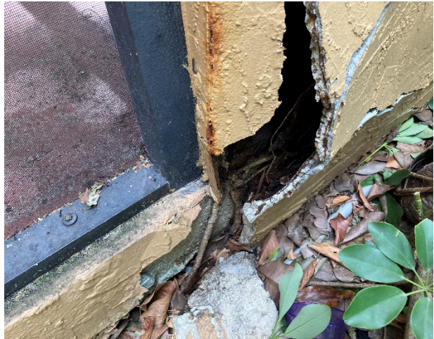
Photograph 4: Unit 105. Opening in the exterior wall
