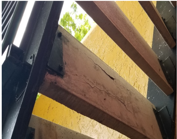
Photograph 10: Concrete steps cracking
