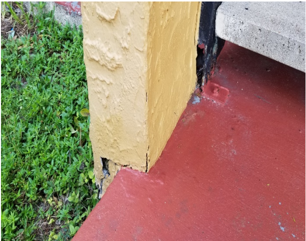
Photograph 9: Opening in the exterior wall
