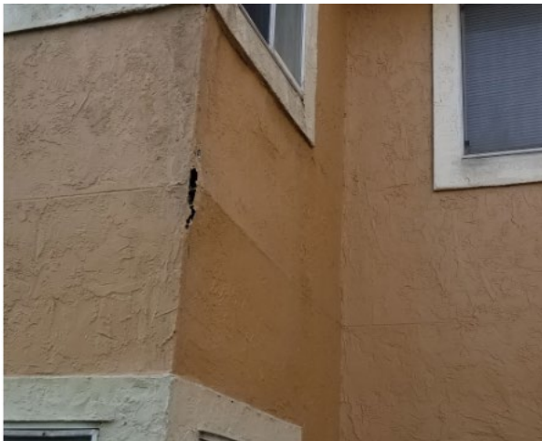
Photograph 11: Opening in the exterior wall
