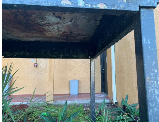
Photograph 14: Common areas staircase landing and columns
