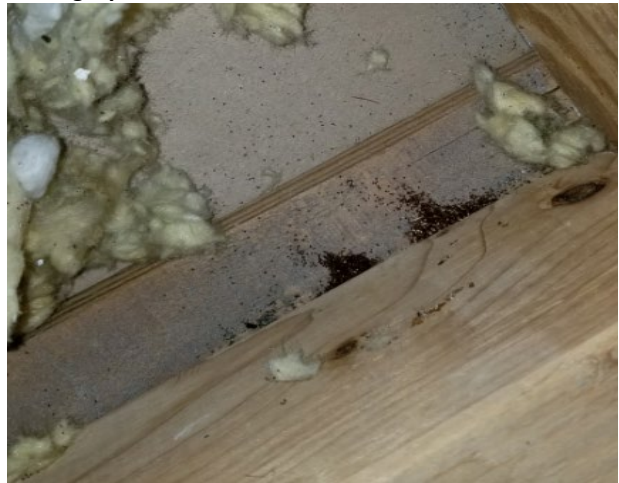
Photograph 6: Termite Infestation
